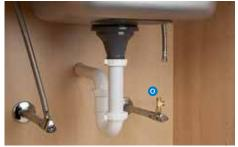
Attach threaded ends of supplied brass tee to the cold water supply line and shutoff valve; tighten using an adjustable wrench.
